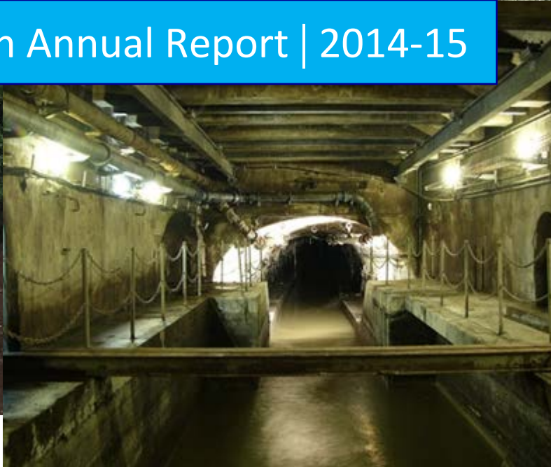
Underground sewers, Paris, France
